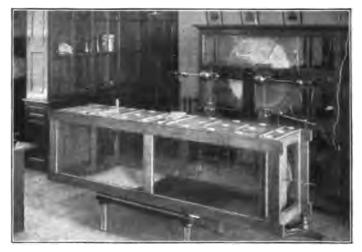
GLASS BOX USED TO DEMONSTRATE THAT MOISTURE FLOWS FROM THE POSITIVE TO THE NEGATIVE POLE.
